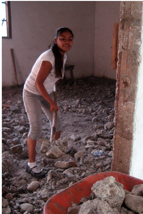
Removing the old cement floor for Aj Awinel's new library
